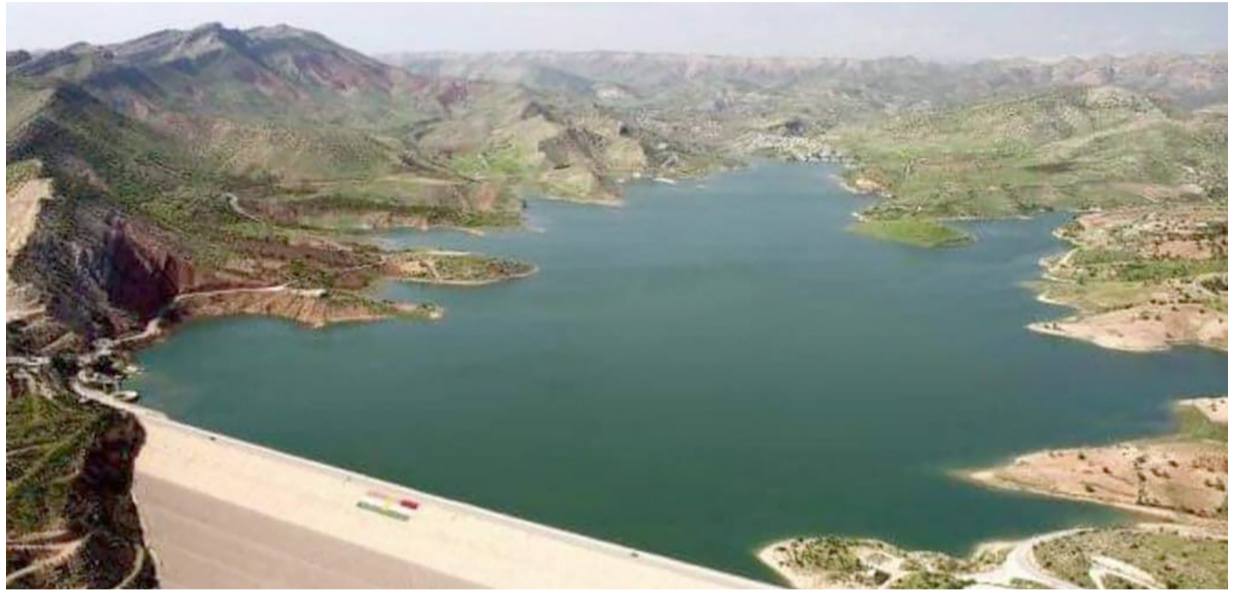
A view of the Duhok dam.
